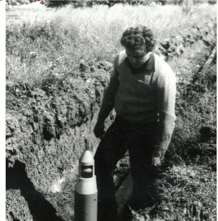
Fig.2c Underground distribution pipeline with a large movable riser \Phi 150 for simultaneous delivery of 30-35 l sec -1 to 30-40 furrows . Such a riser delivers water consequently to the left & right and covers a 100m strip of land, or 20 to 40 dka irrigated area. Flexible distribution pipeline diameter could be \Phi 200 .
